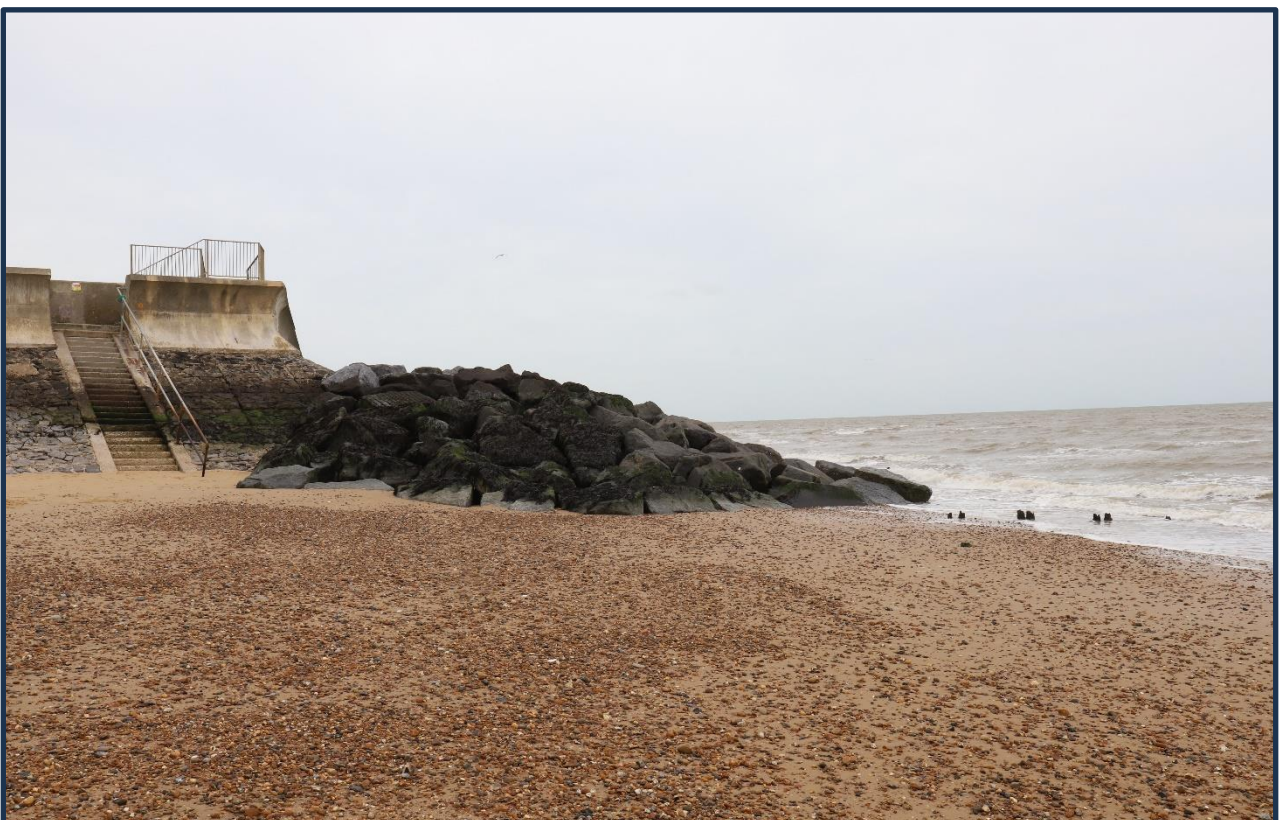
Photo 6: View of recent coastal defence scheme looking north from the foreshore
